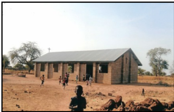
School building complete with roof!
